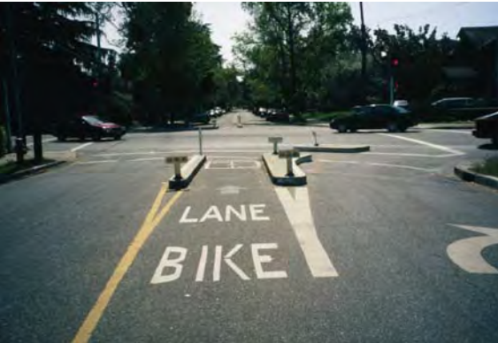
Figure 5.6 Bicycle activated signal
