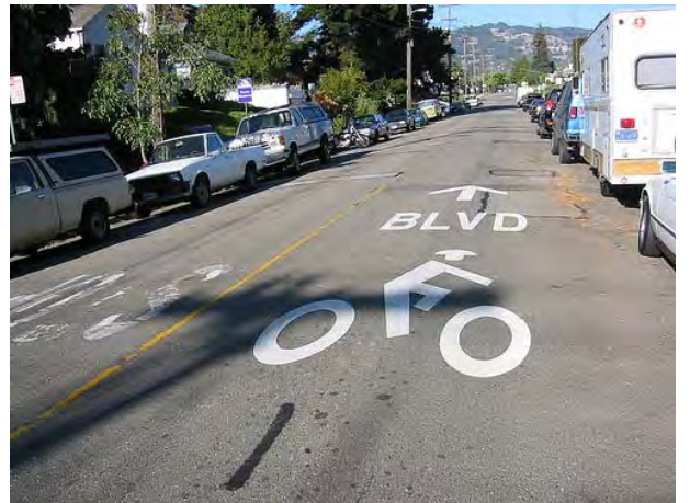
Figure 5.7 Large pavement markings
