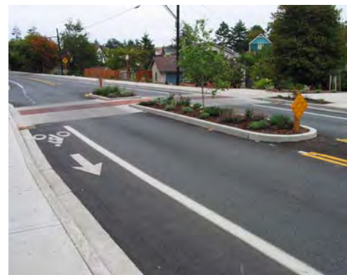
Crosswalk and Median Refuge
