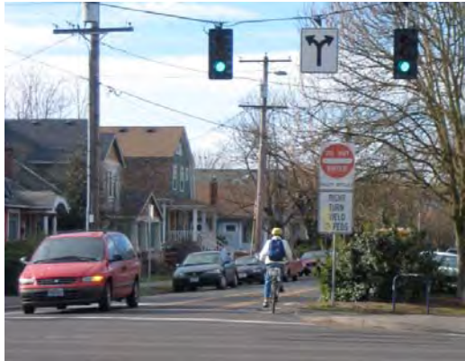
Figure 5.13 A signalized partial non-motorized crossing only allows motorists to exit the bikeway while cyclists may continue through.
