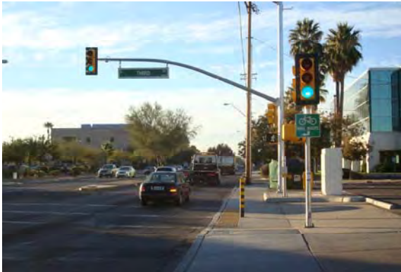
Figure 5.19 A two-way bicycle side path and signalized crosswalk at East Third Street and North Alvernon Way.
