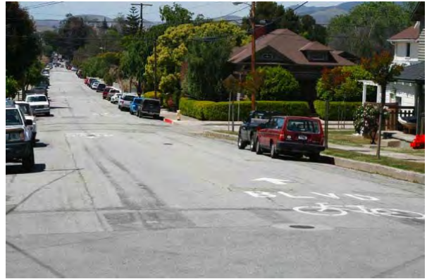
Figure 5.1 Pavement markings and signage identify the street as a bicycle boulevard.
