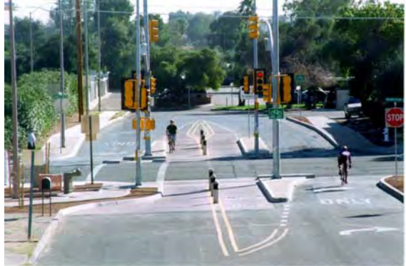
Figure 5.21 A TOUCAN signal at North Country Club Road and East Third Street requires motorists to turn right while a bicycle signal head allows through movements by cyclists
