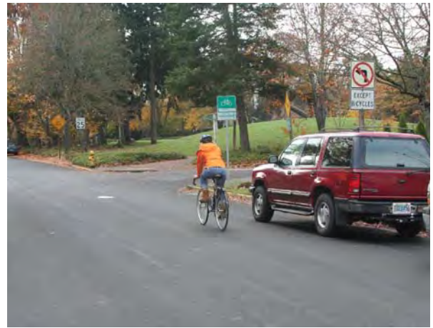
Figure 5.16 Speed tables, wayfinding signage, pavement markings, and non-motorized only crossings work together to create the bicycle boulevard
