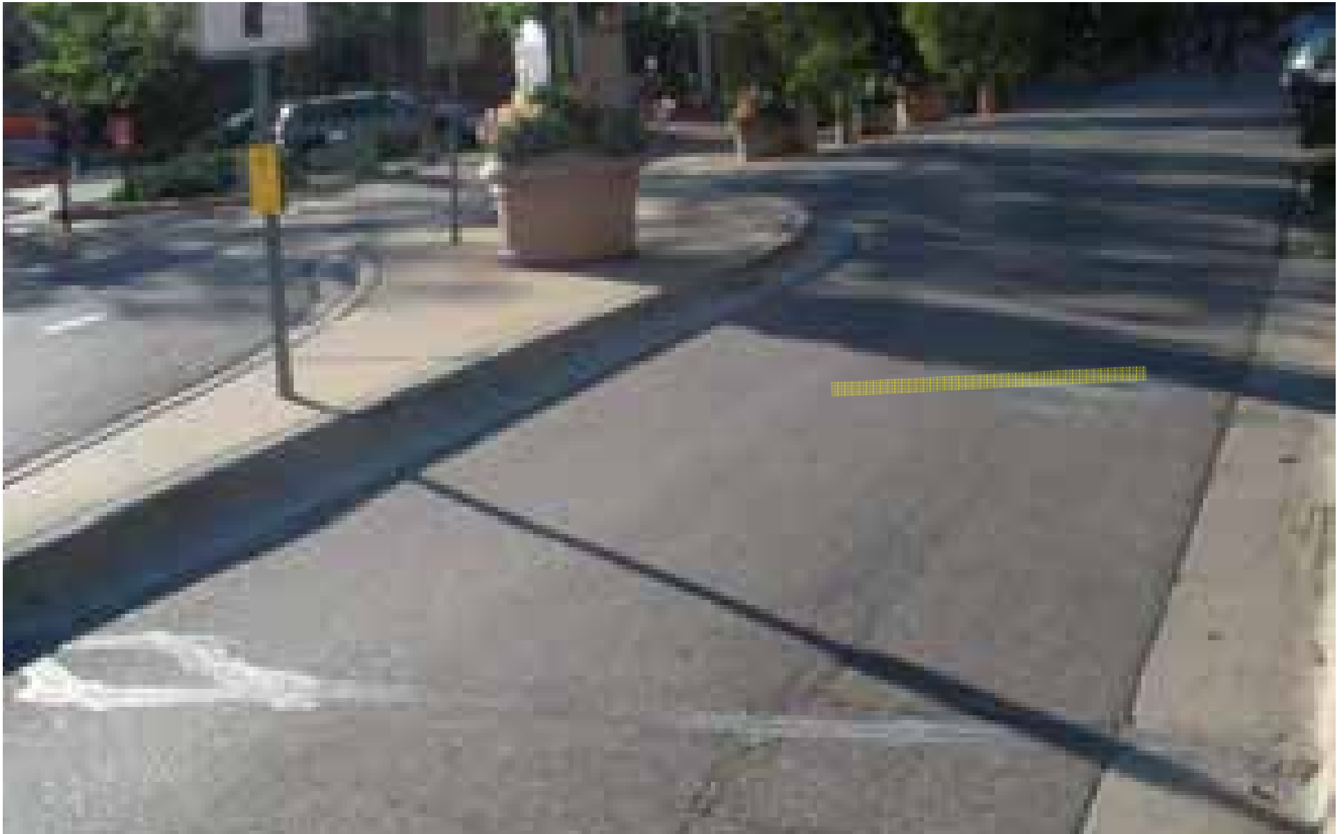
Inductive loop counters in vehicle lane
