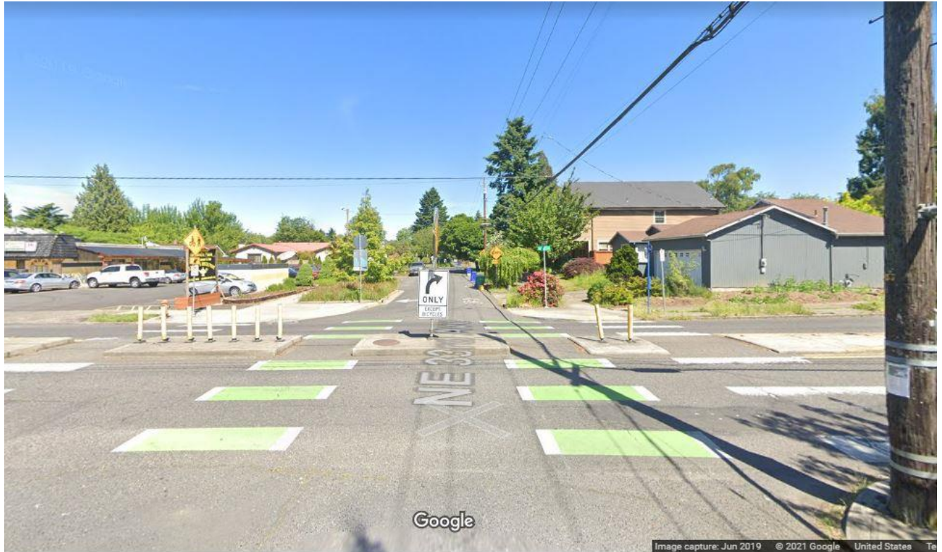
Figure 1: Typical intersection with cross-bike pavement markings.
